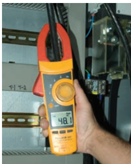
Actual Amp Load Measured Inside Panel with Amp Meter: 48.1
