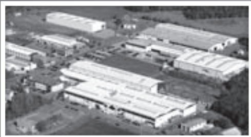
Headquarter Bad Marienberg | Germany
