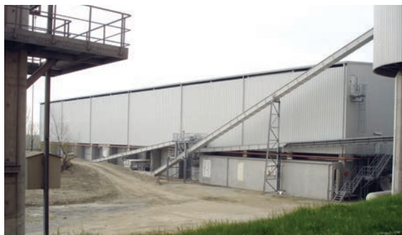
Drag Chain Conveyor installation for long distances.
